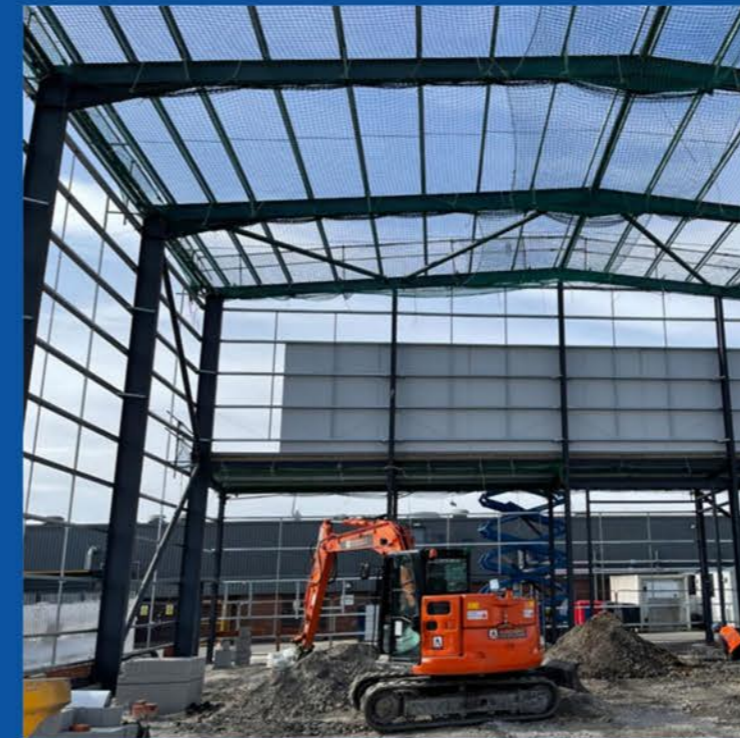
FACTORY MAINTENANCE SHED Barbil, Odisha
