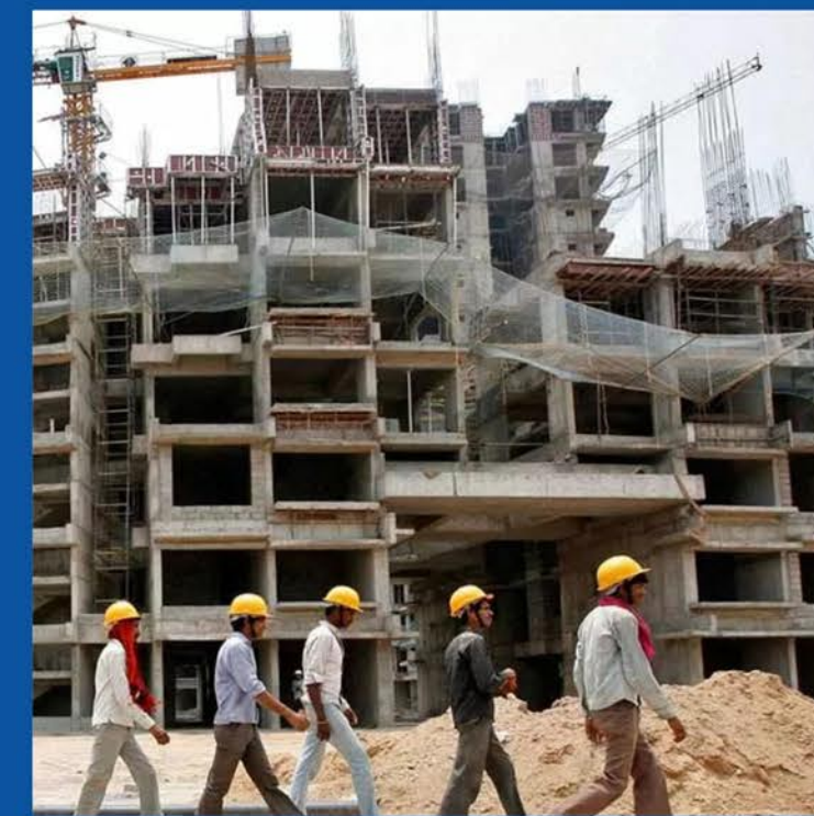
CONSTRUCTION OF G+3 RESIDENTIAL BUILDING
