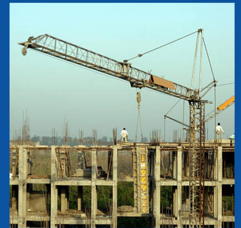
CONSTRUCTION OF B+G+12 RESIDENTIAL BUILDING
